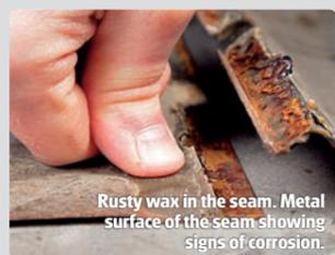
Rusty wax in the seam. Metal surface of the seam showing signs of corrosion.
